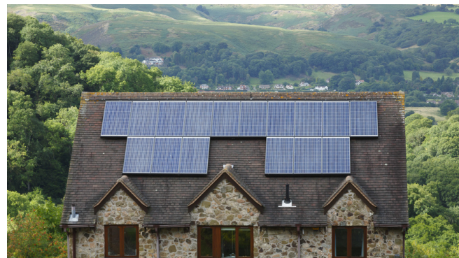
Solar panels on roof
